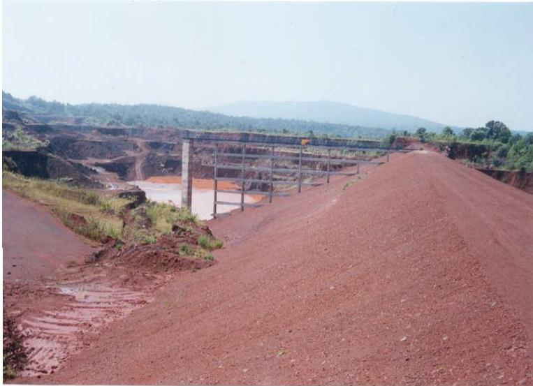
The Slime from the ore washing plant is separately stored in zero discharge slime dam for possible future use.
