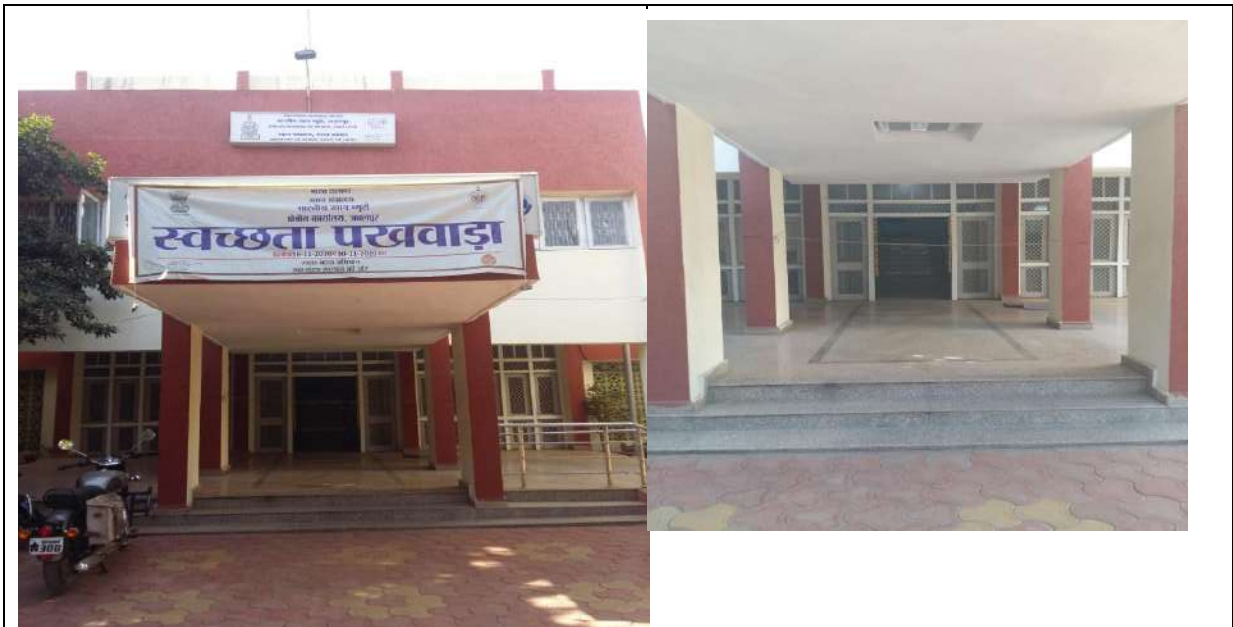
A view of Entry of IBM office indicating cleaning of office building
