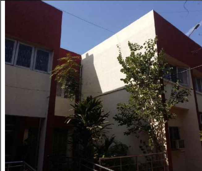
A view of office building after cleaning
