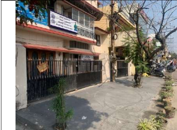
Cementing of Pathway of Dehradun RO
