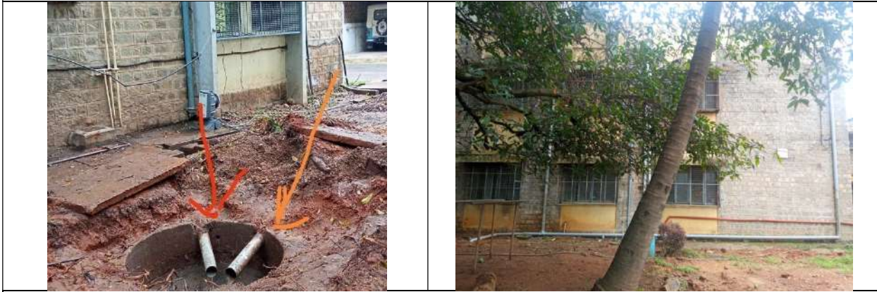
Repairing of Rainwater Harvesting System at Bangalore
