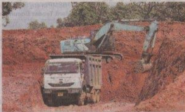
Taking off: After limestone, most of the blocks are those of iron ore. (Picture for representational purpose only).
